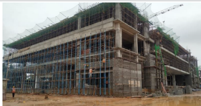
Figure 2. Progress at RAK's new manufacturing facility in Bengaluru, India
